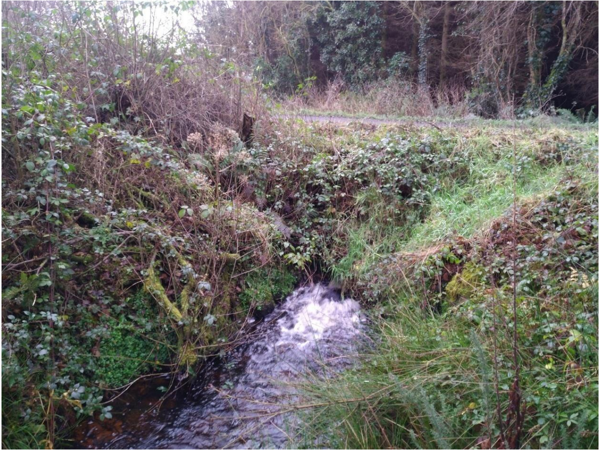
Figure 21 View of Downstream Elevation of Structure No. 7
