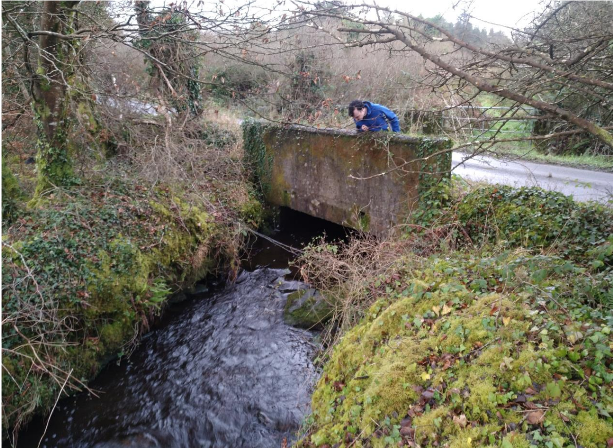
Figure 25 View of Downstream Elevation of Structure No. 8
