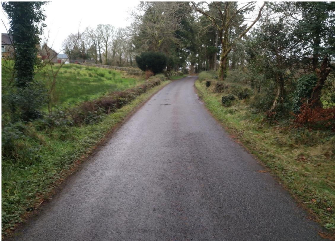
Figure 9 View of Road Carriageway above Structure No. 2
