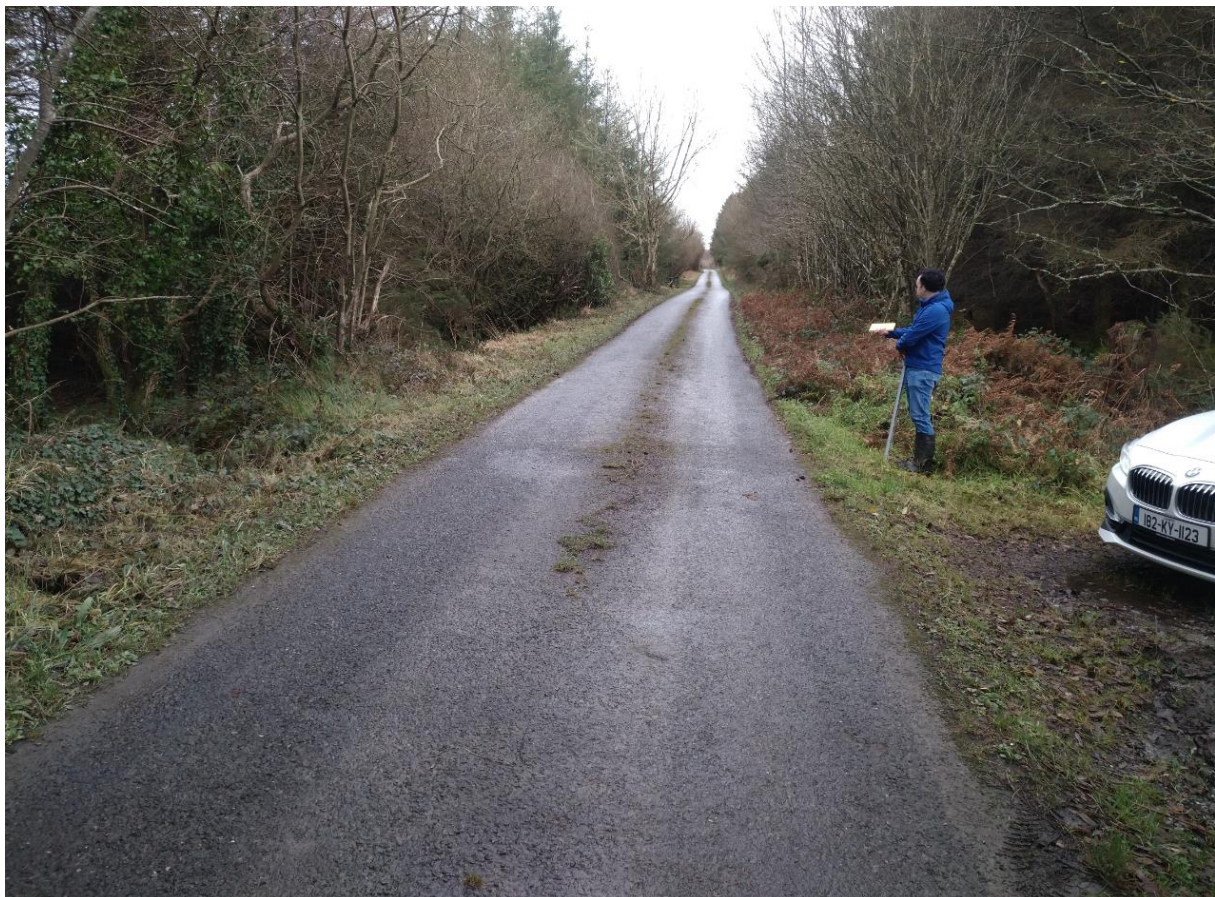
Figure 17 View of Road Carriageway above Structure No. 5
