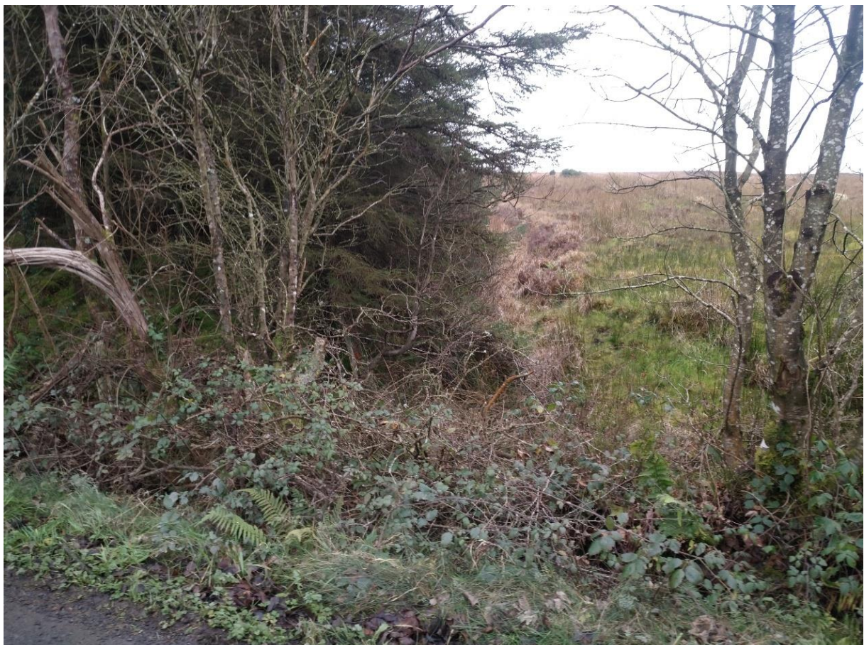
Figure 19 View Upstream at Structure No. 6
