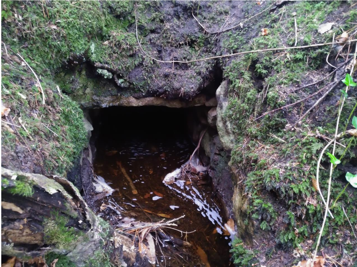
Figure 8 View of Downstream Elevation of Structure No. 2
