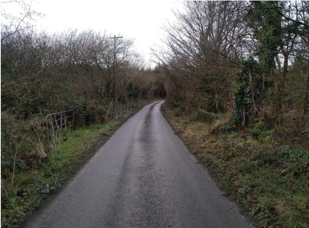
Figure 28 View of Road Carriageway above Structure No. 8
