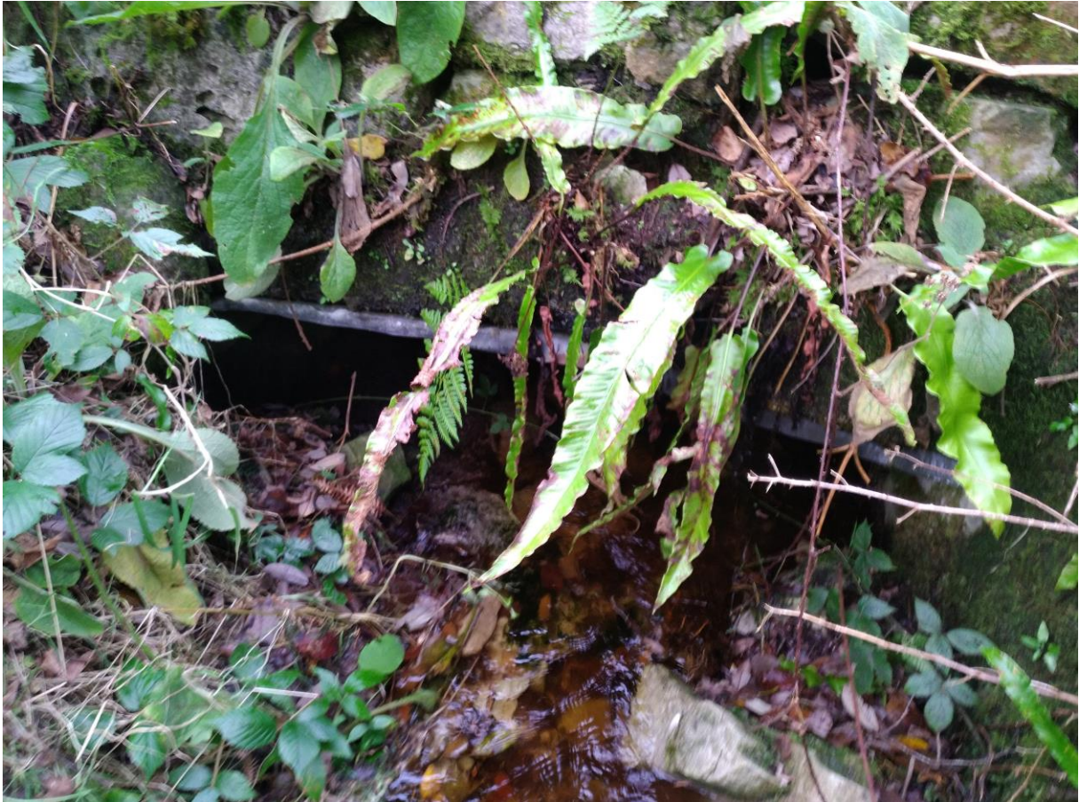
Figure 14 View of Upstream Elevation of Structure No. 5
