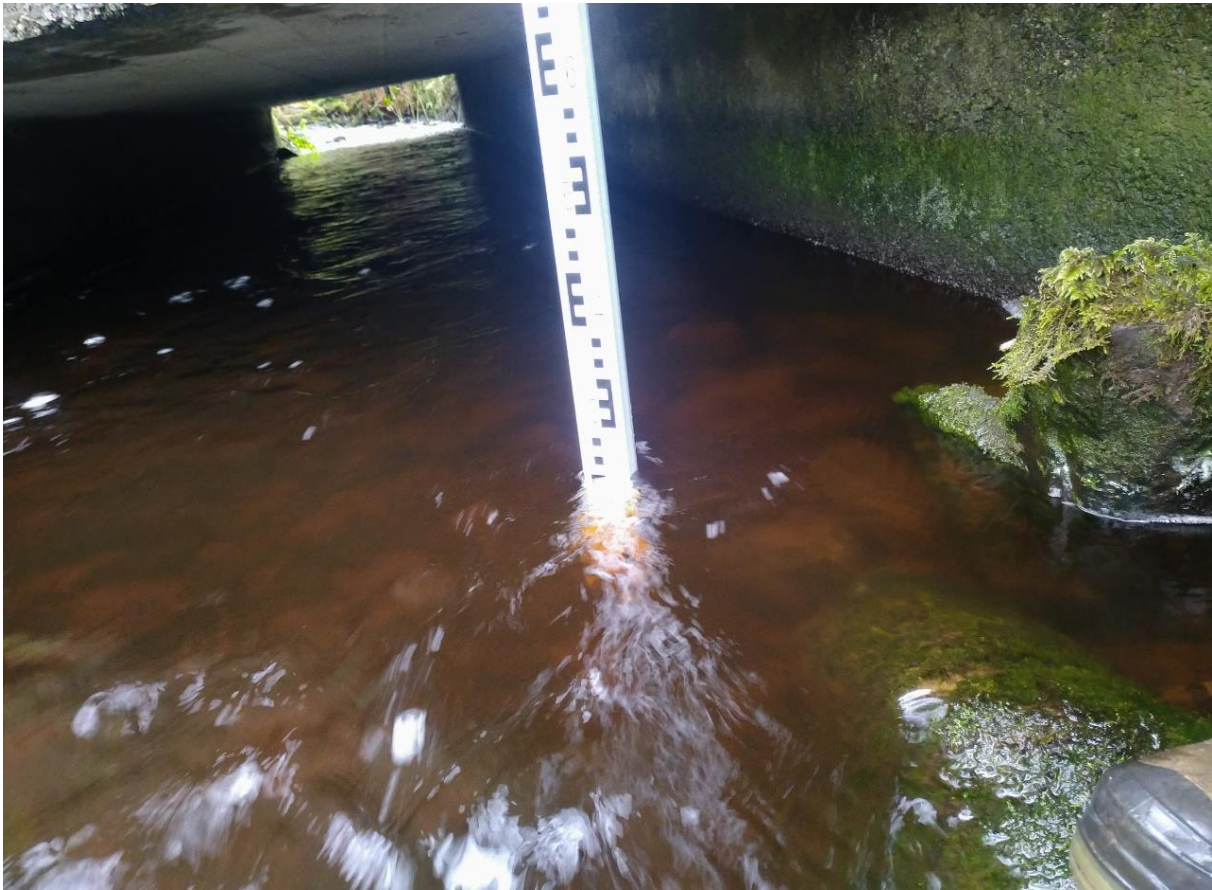
Figure 27 View of Channel within Structure No. 8
