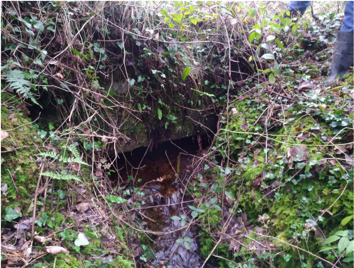
Figure 16 View of Downstream Elevation of Structure No. 5
