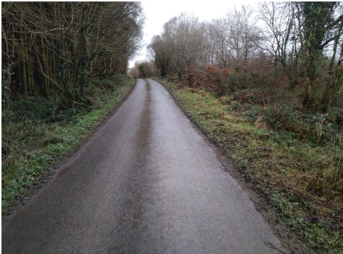
Figure 24 View of Road Carriageway above Structure No. 7
