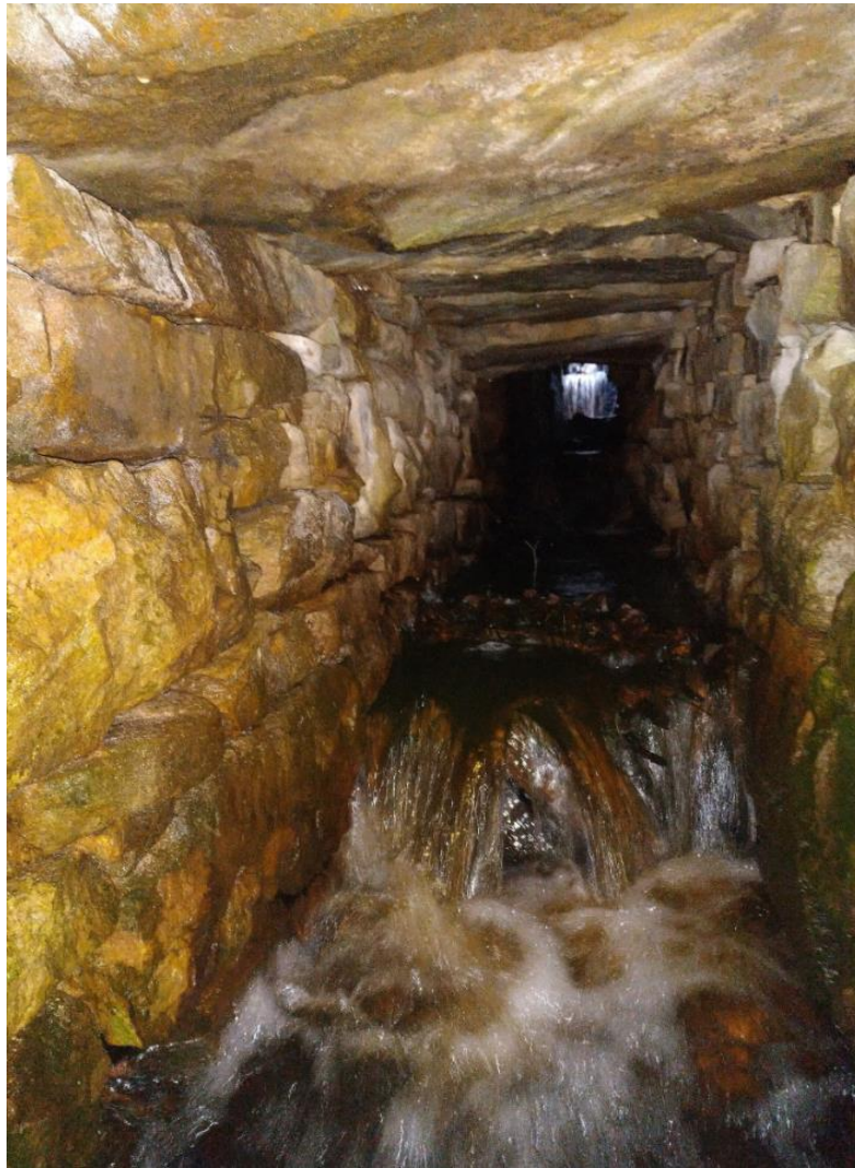
Figure 5 View inside Span 2 of Structure No. 1
