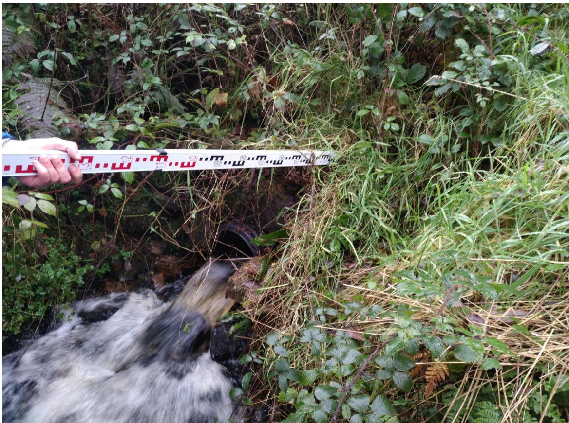
Figure 22 View of 300mm \varnothing CorriPipe within Structure No. 7 at Downstream Elevation
