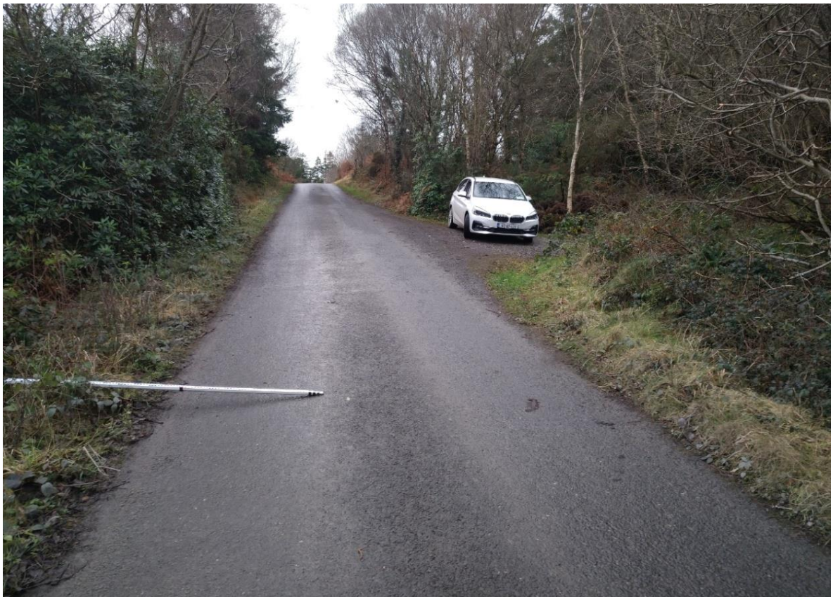
Figure 11 View of Road Carriageway above Structure No. 3
