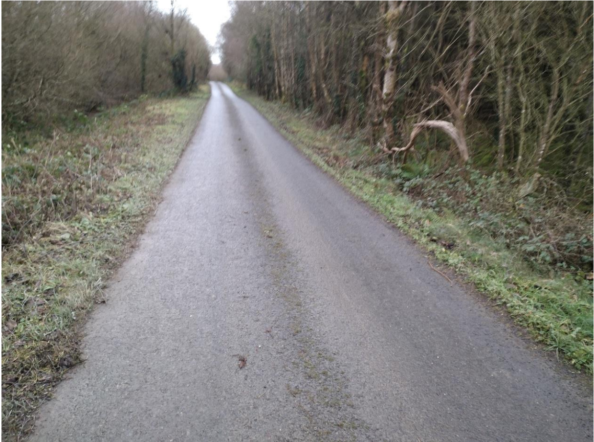
Figure 20 View of Road Carriageway over Structure No. 6
