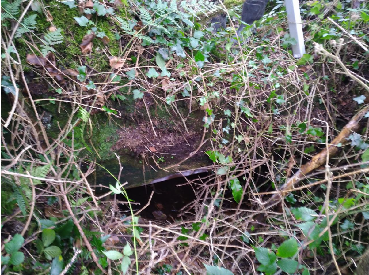
Figure 12 View of Downstream Elevation of Structure No. 4
