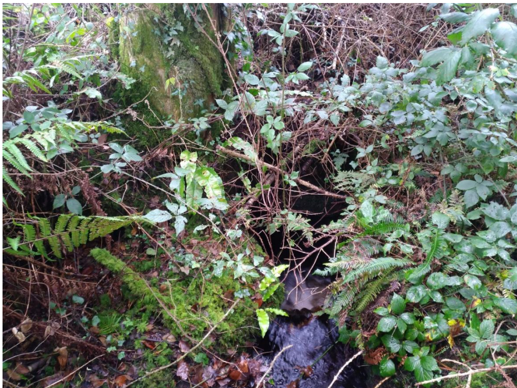
Figure 6 View of Upstream Elevation of Structure No. 1
