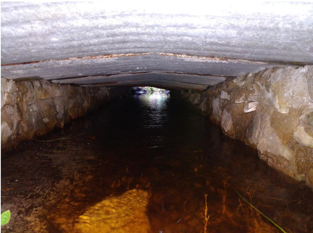
Figure 15 View inside Channel of Structure No. 5
