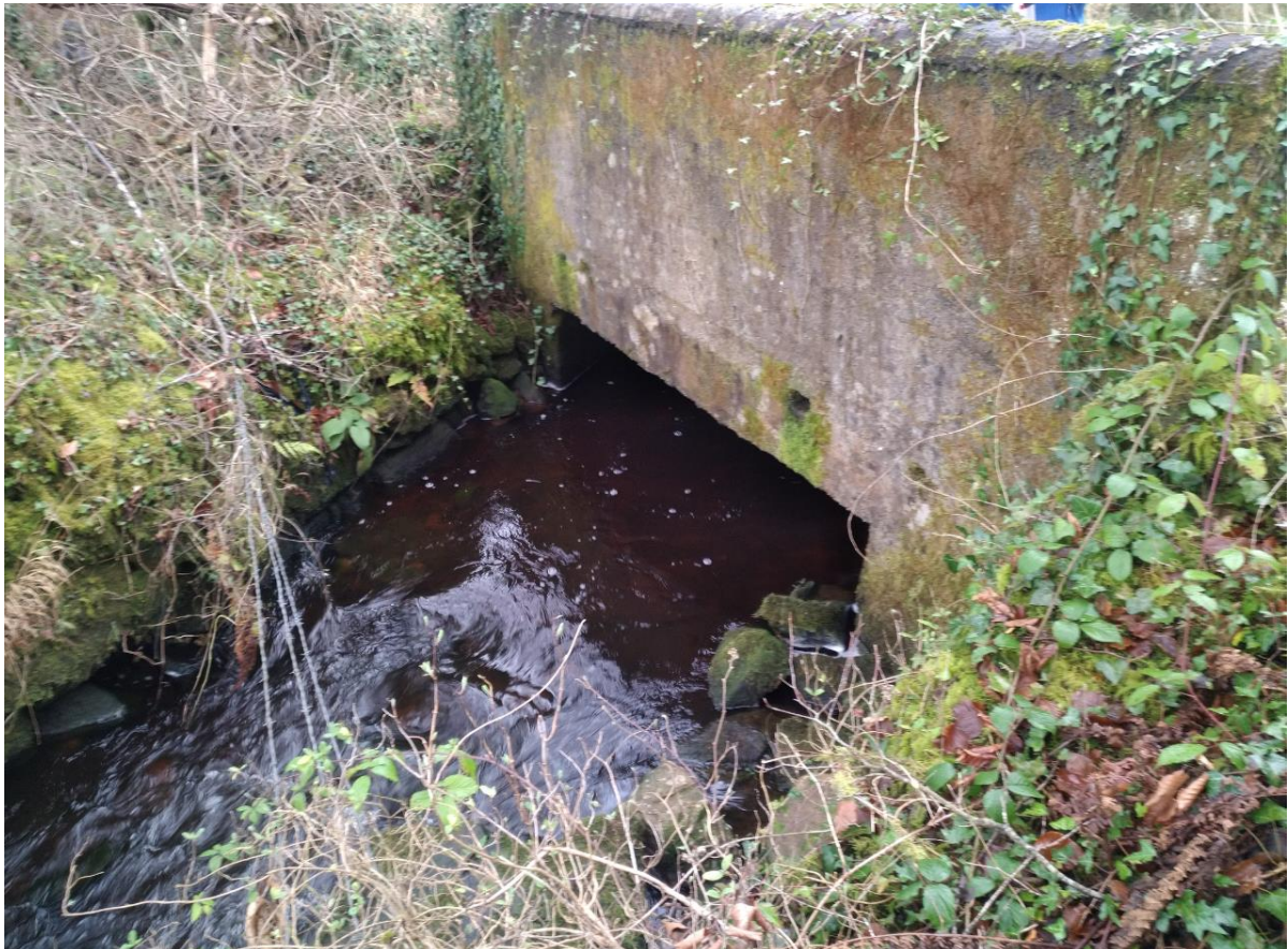
Figure 26 View of Downstream Elevation of Structure No. 8
