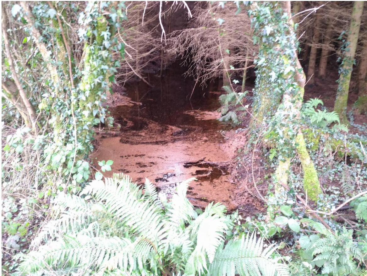
Figure 23 View Upstream of Structure No. 7
