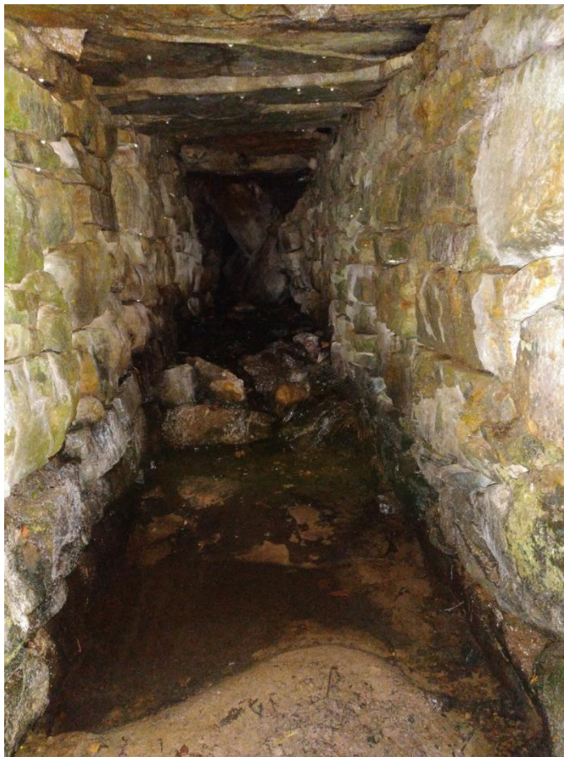
Figure 4 View inside Span 1 of Structure No. 1
