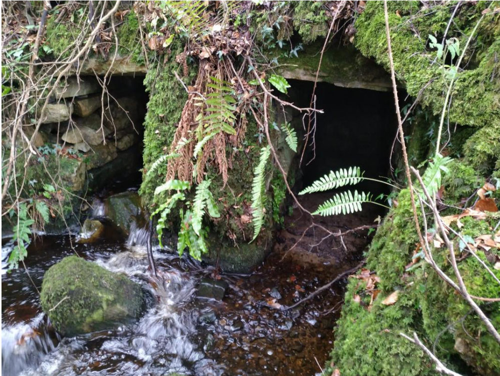
Figure 3 View of Downstream Elevation of Structure No. 1
