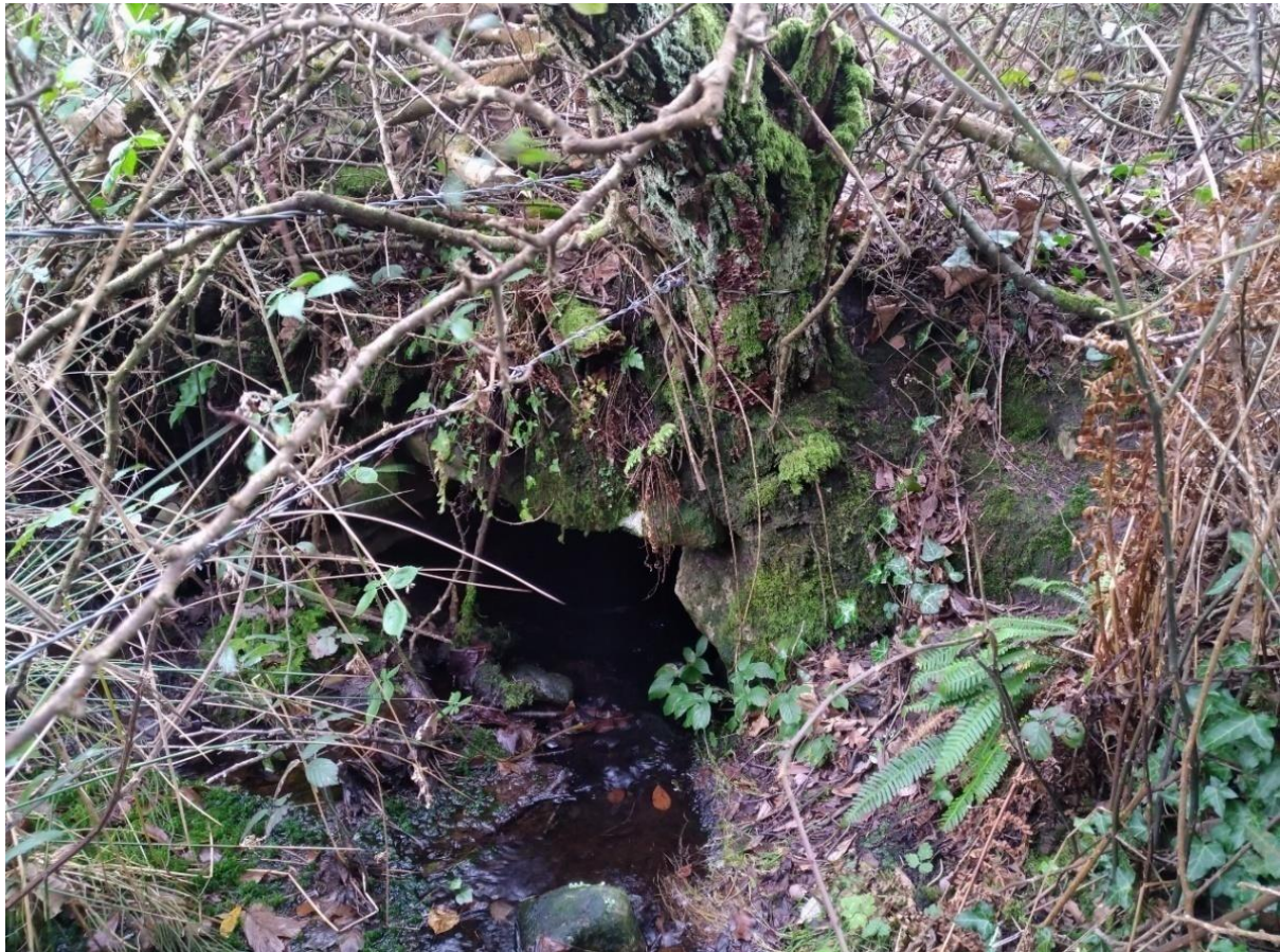
Figure 18 View of Upstream Elevation of Structure No. 6
