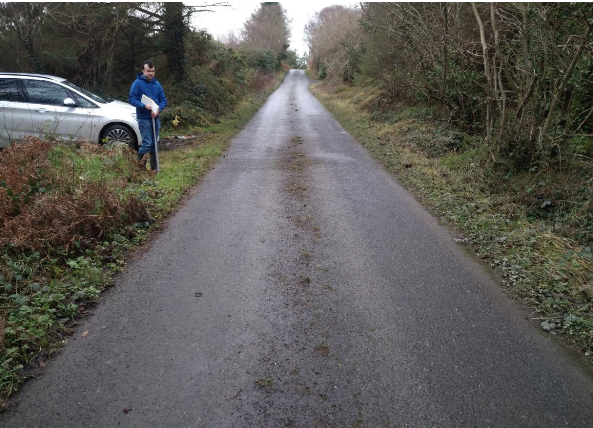
Figure 13 View of Road Carriageway above Structure No. 4
